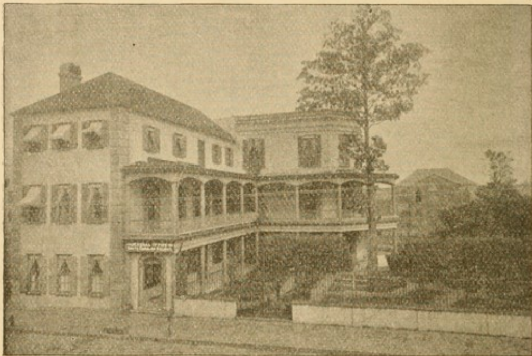
The South Carolina Railway Offices.
