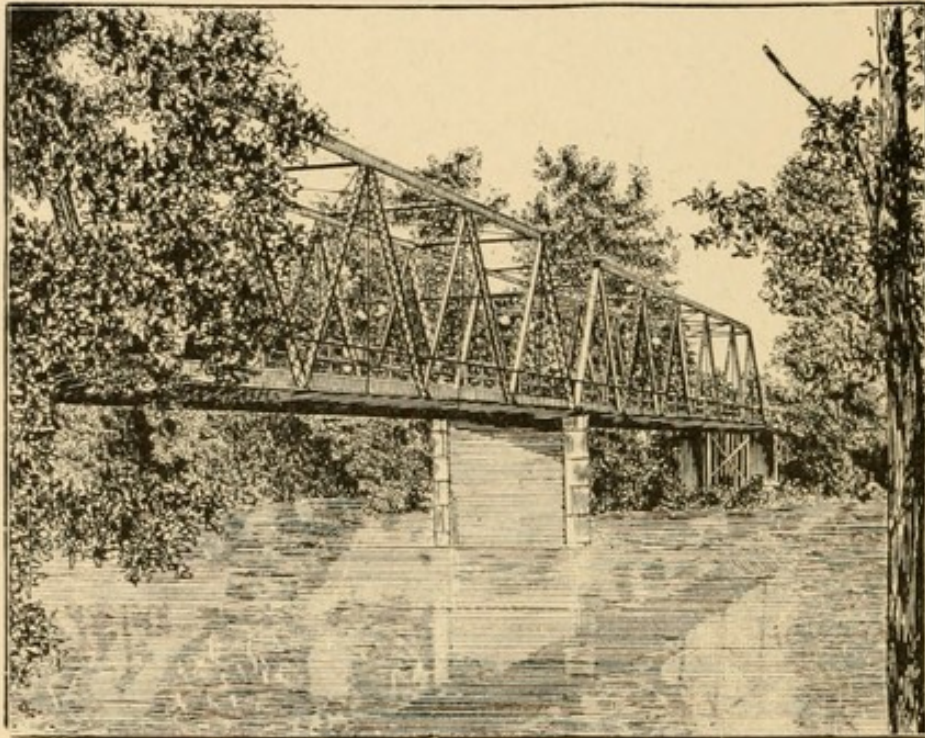
Bridge over the Wateree River.
