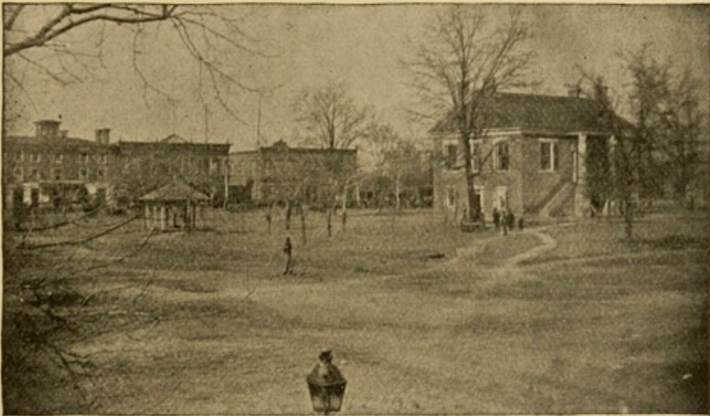
Central Hotel, Opera House, Masonic Hall and Court House.
