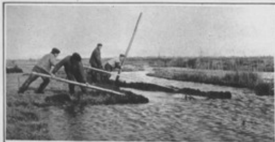
THE DUTCHMAN'S WAY OF BUILDING HOUSES IN MARSHY PLACES (1) Cutting the peat soil into long strips, which are (2) covered by boats to the place where the house is to be built.
