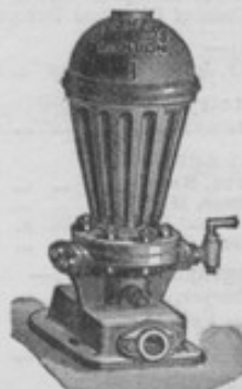
WARNER'S IMPROVED HYDRAULIC RAMS, WITH NEWLY-DESIGNED VALVES AND AUTOMATIC ARRANGEMENTS, IN VARIOUS SIZES.
