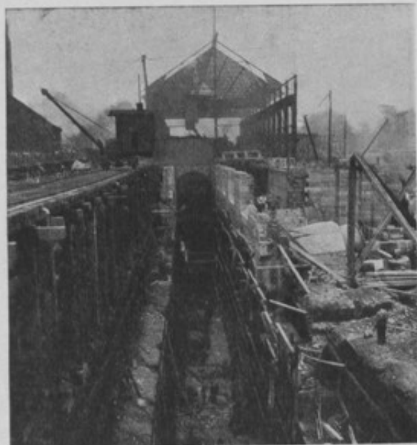
FIG. 2.—Power House of Canadian Niagara Power Co., being erected over the wheel-pit.
