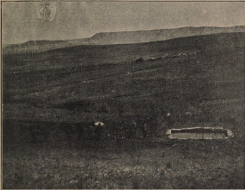
(7) Surface pond, artificially formed, to collect water from springs. The water is pumped from the pond into the water-carts for conveyance to camps. (Newcastle.)
