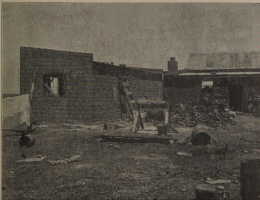
(35.) Surface well, feeding an aerated water factory at Modder River. Note insanitary surroundings of the well and the absence of any protection of soil, &c., to prevent surface water percolating into the well.
