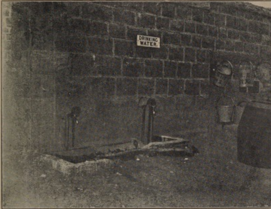
(14.) Water laid on to taps from different sources at railway station, Standerton. The tap on left yields what is practically sewage; the tap on the right yields unpurified river water collected above the town.
