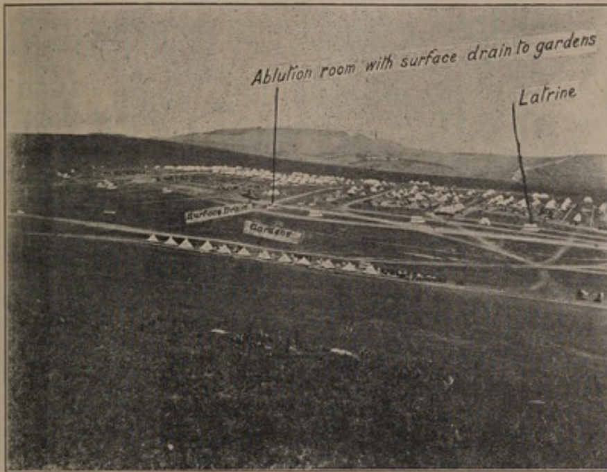
(40.) Camps of Cavalry and Artillery at Mooi River; showing horse lines outside and below men's lines; ablution room and latrines, below the horse lines; and gardens at the bottom of the slope, irrigated by ablution-room water.
