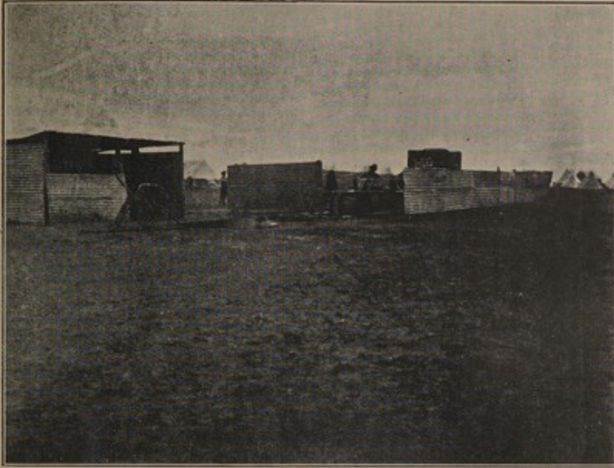
(20.) Corrugated-iron sheds. Concrete channel to large concrete sump; but no concreting of soil within enclosure. The covered shed contained wooden tubs for body baths, placed on unprepared surface soil. (Kroonstad.)
