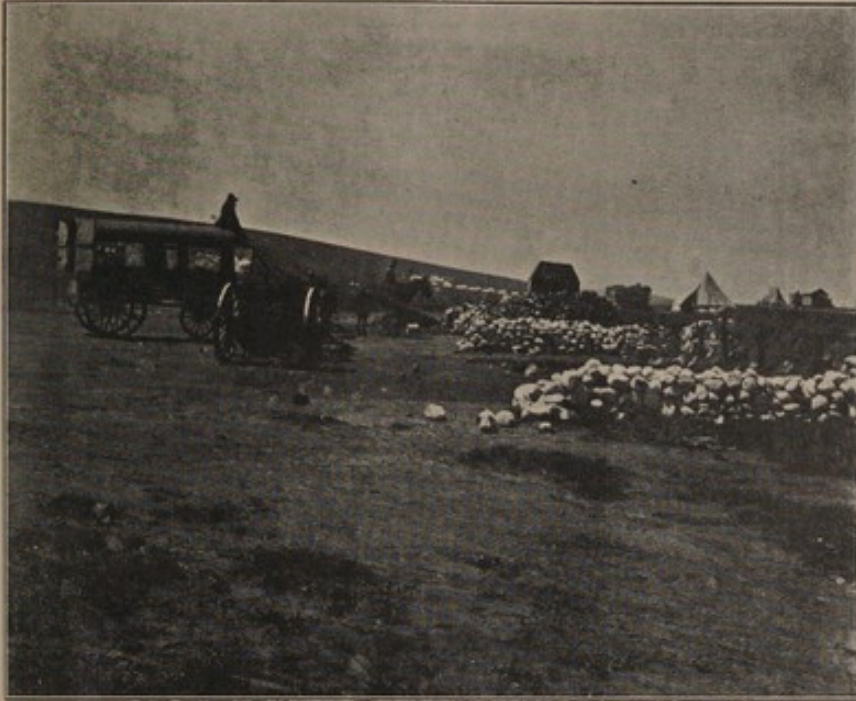
(30.) Incinerator for dry refuse, also refuse carts. (Mooi River camps.)
