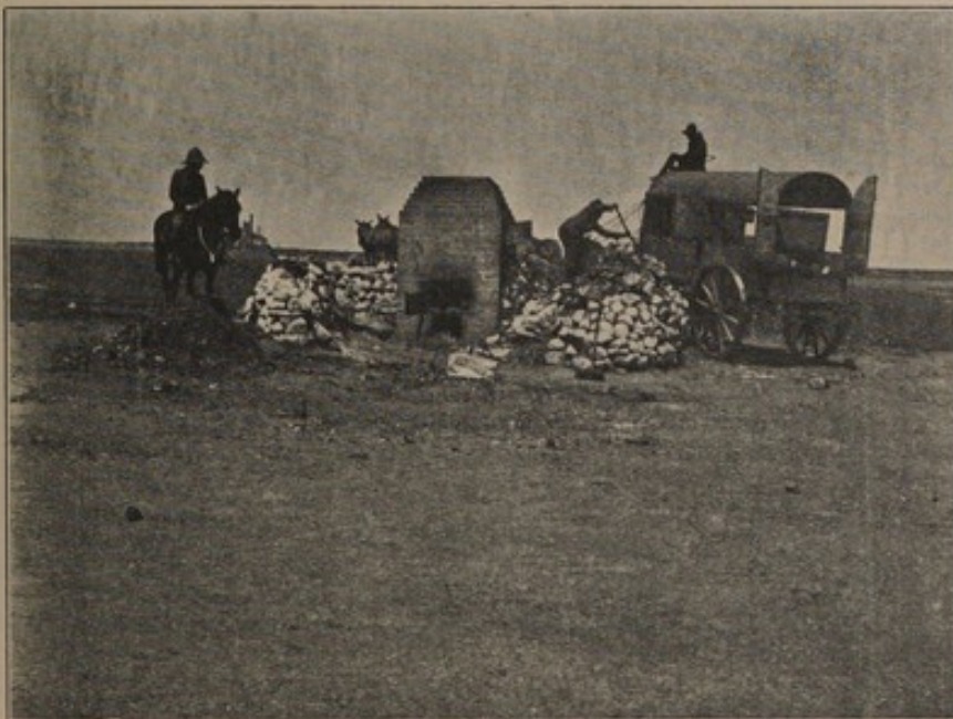
(31.) Incinerator for dry refuse, showing stone enclosure, stokehole, and aperture for raking refuse into furnace. (Mooi River camps.)
