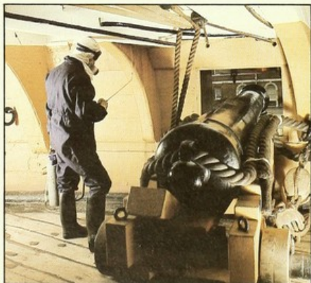
Protecting with 'Coopex' the oak timbers of Nelson's flagship, 'HMS Victory'
