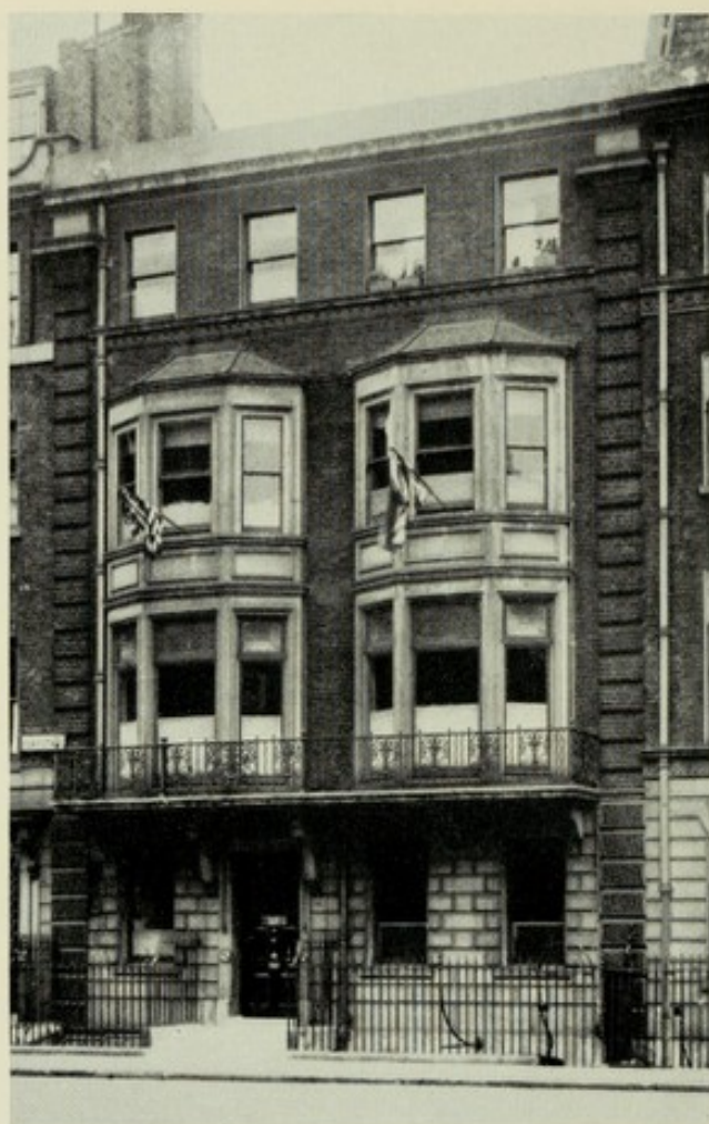
Fig. 4 10 Henrietta Street (now Henrietta Place), London, W.1
