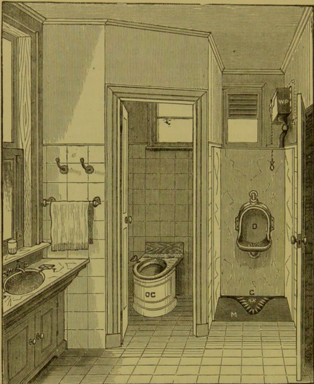
FIG. 282.—View of a Billiard-room Lavatory; or Door-action Urinal, Water-closet, and Lavatory.
