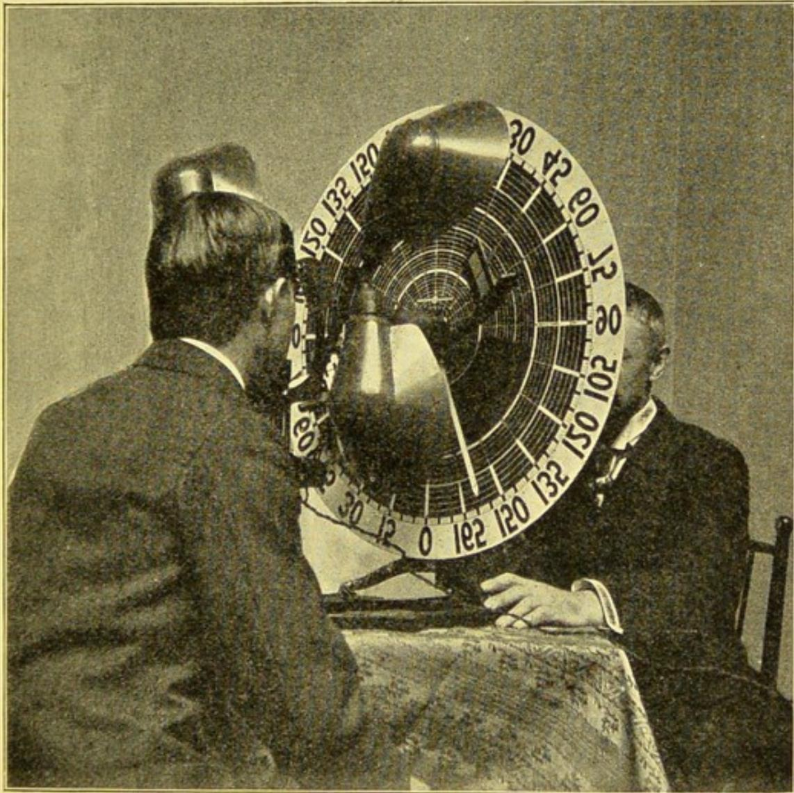
FIG. 13.—THE OPHTHALMOMETER IN USE
