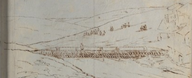
Bridge across a ravine resting on Cannibal barrels with their heads removed for water to pass through after heavy rains -
