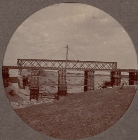
Zand River Bridge.
