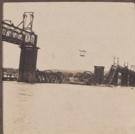
Aerial Bridge, Norvals Pont.
