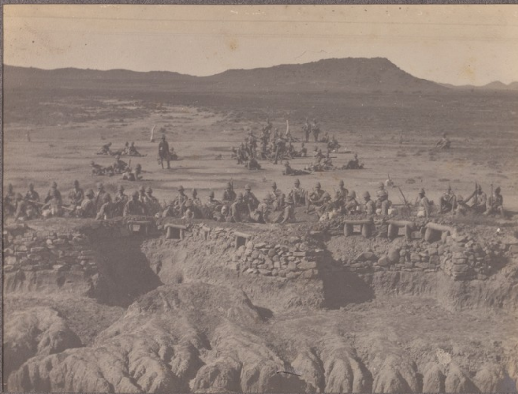
Suffolk trenches cut out of the side of a spruit.
