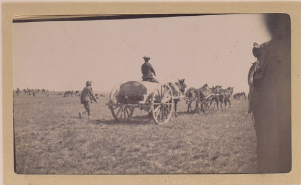
Water Cart (Drinking Water)
