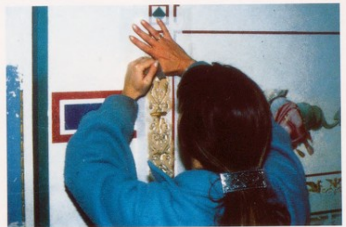
A substantial investment in time and money was needed to repair the damage done to the frescos. Sheppard Robson (top), Pauline Plummer (bottom)
