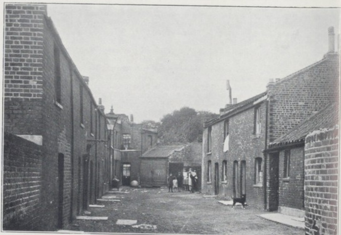
PHOTOGRAPH No. 4.—Conduit Place, NORTHWOLD ROAD AREA.
