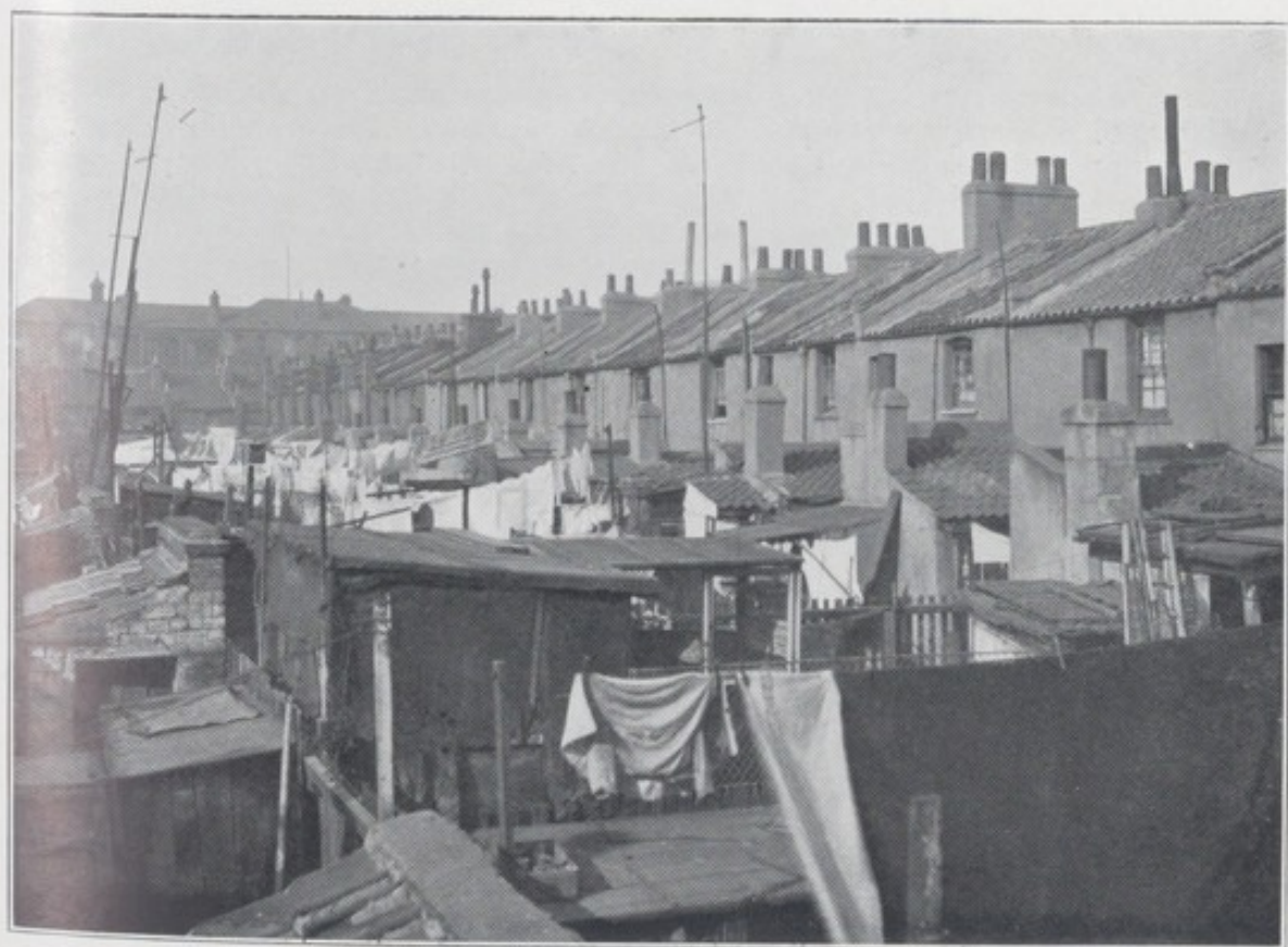
PHOTOGRAPH No. 10.—Back view of houses in College Street, BANISTER STREET AREA.
