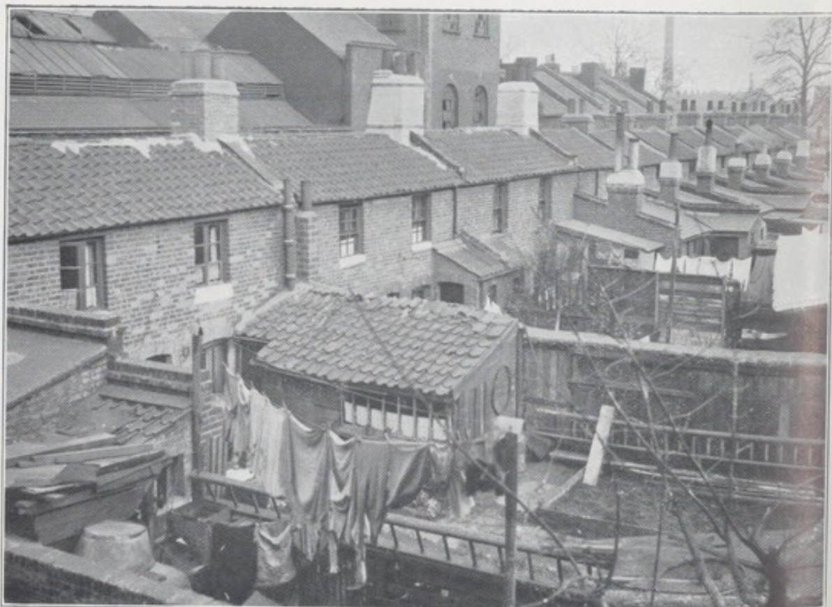
PHOTOGRAPH No. 24.—Backs of cottages in Otley Terrace, OTLEY TERRACE AREA.
