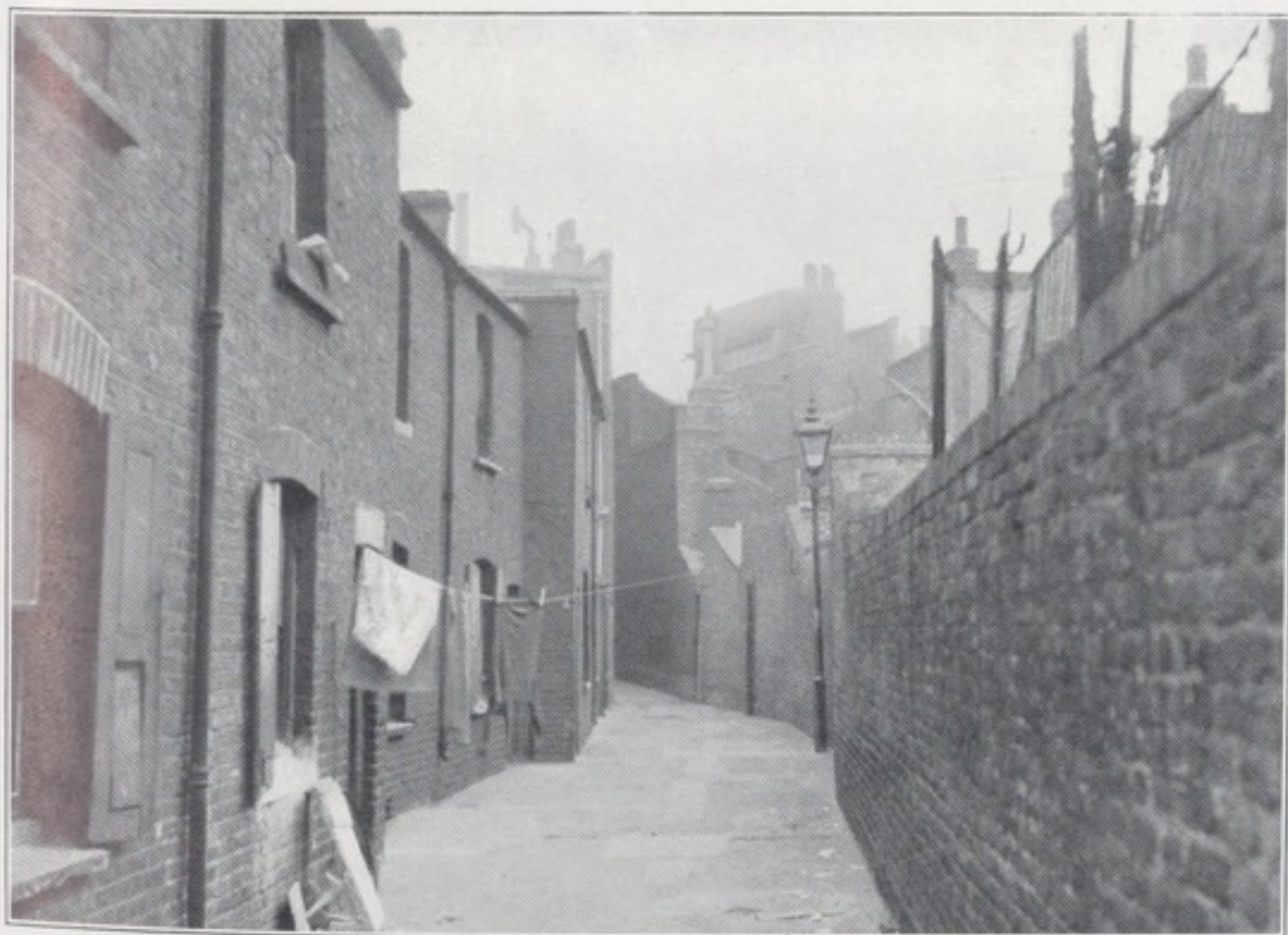
PHOTOGRAPH No. 30.—Queens Court, looking south, QUEENS COURT AREA.
