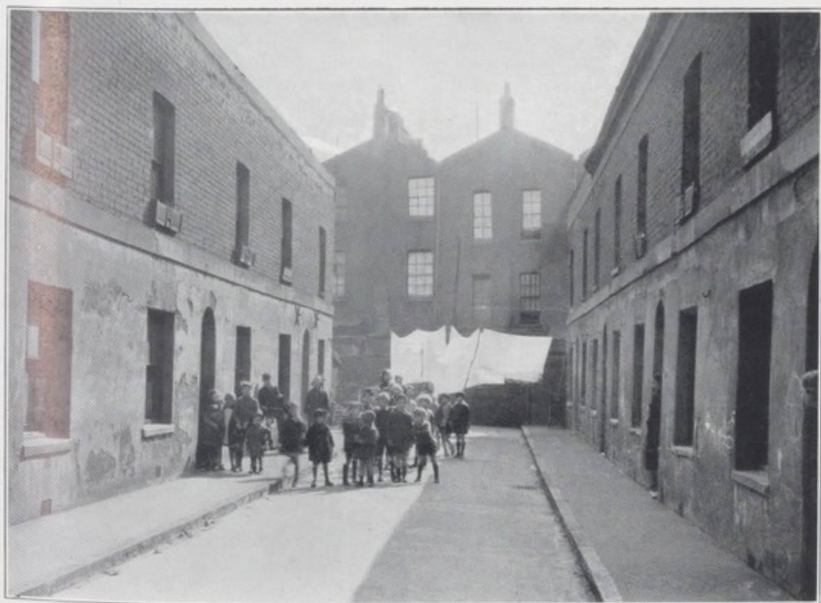
PHOTOGRAPH No. 14.—Front view of Clarence Cottages, CLARENCE TERRACE AREA.
