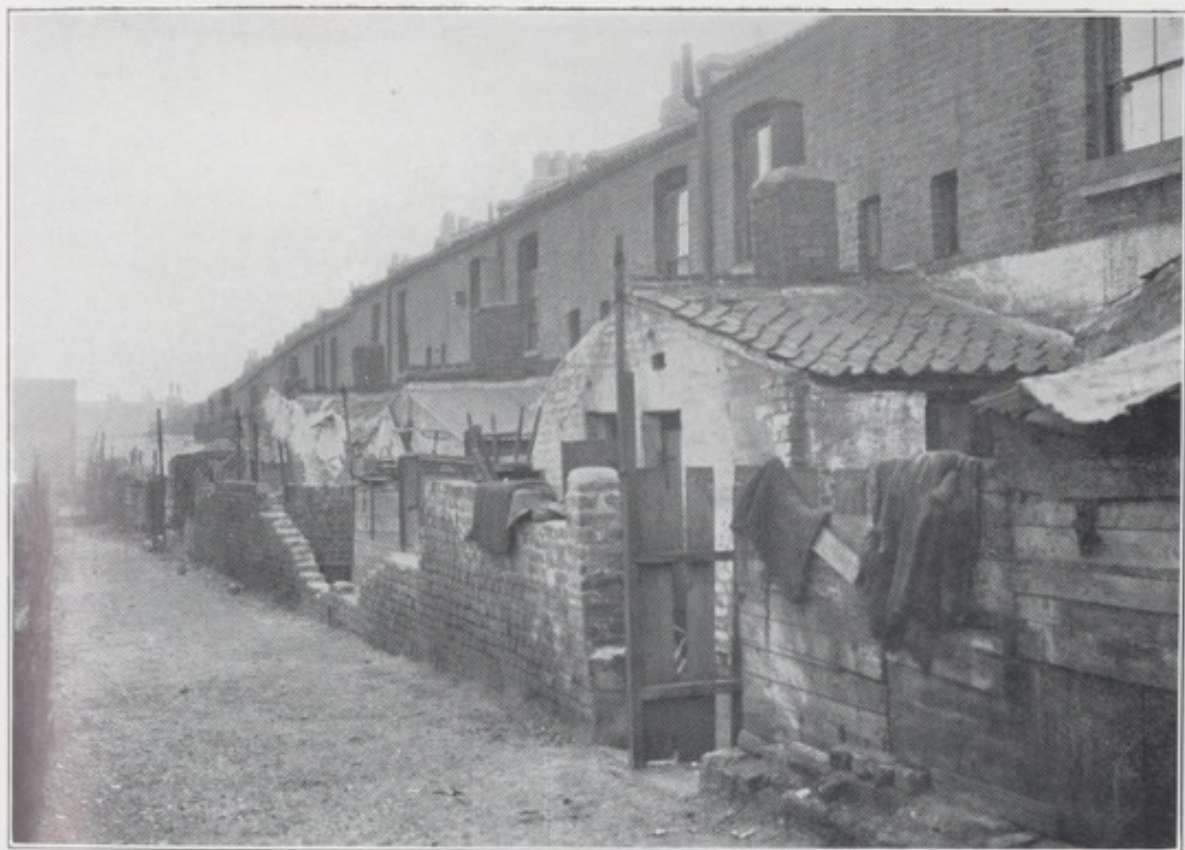
PHOTOGRAPH No. 21.—Back view of Nisbet Street, looking south, NISBET STREET AREA.
