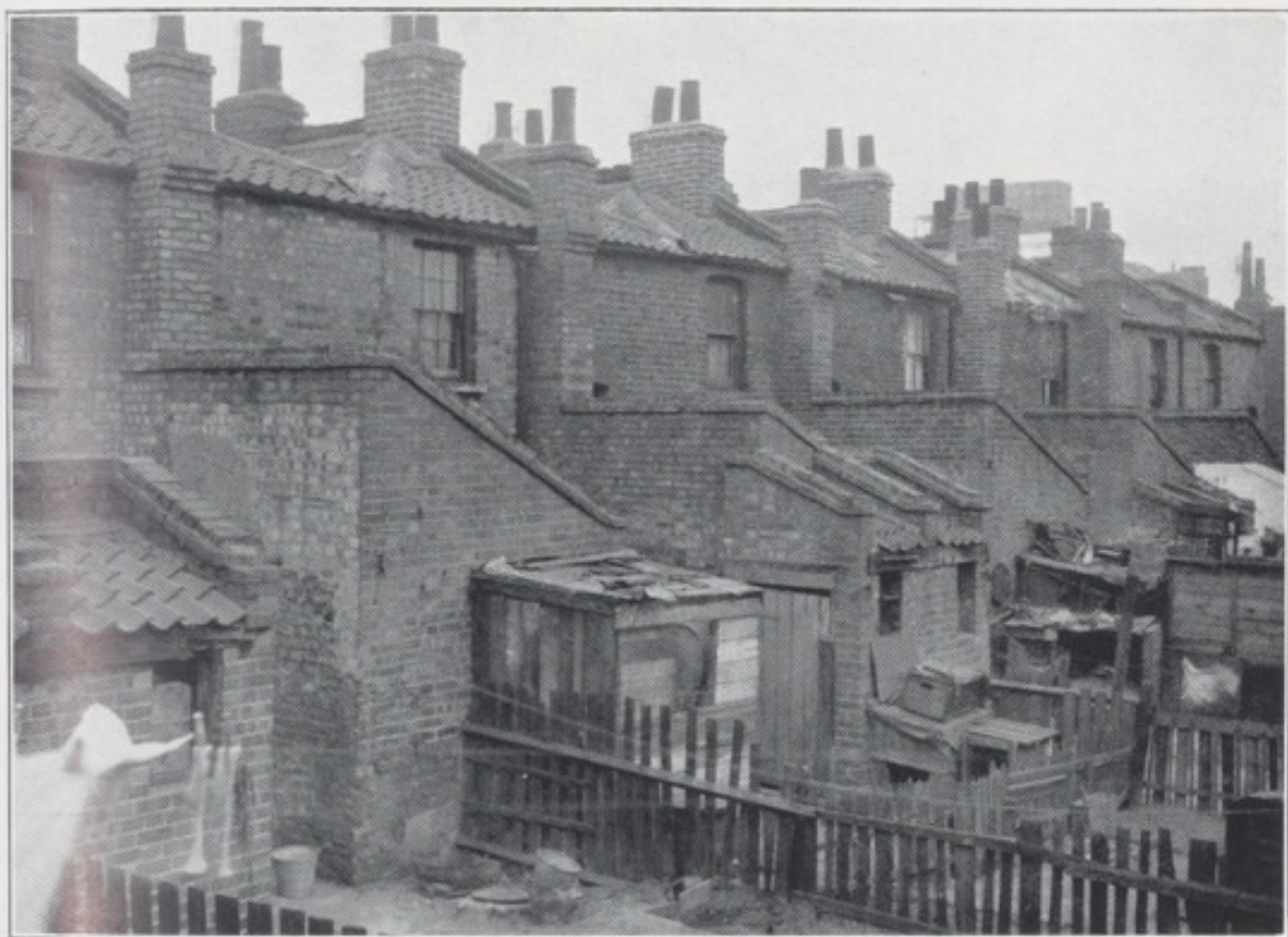
PHOTOGRAPH No. 13.—Backs of south side of Ada Street looking north-east, BROADWAY AREA.
