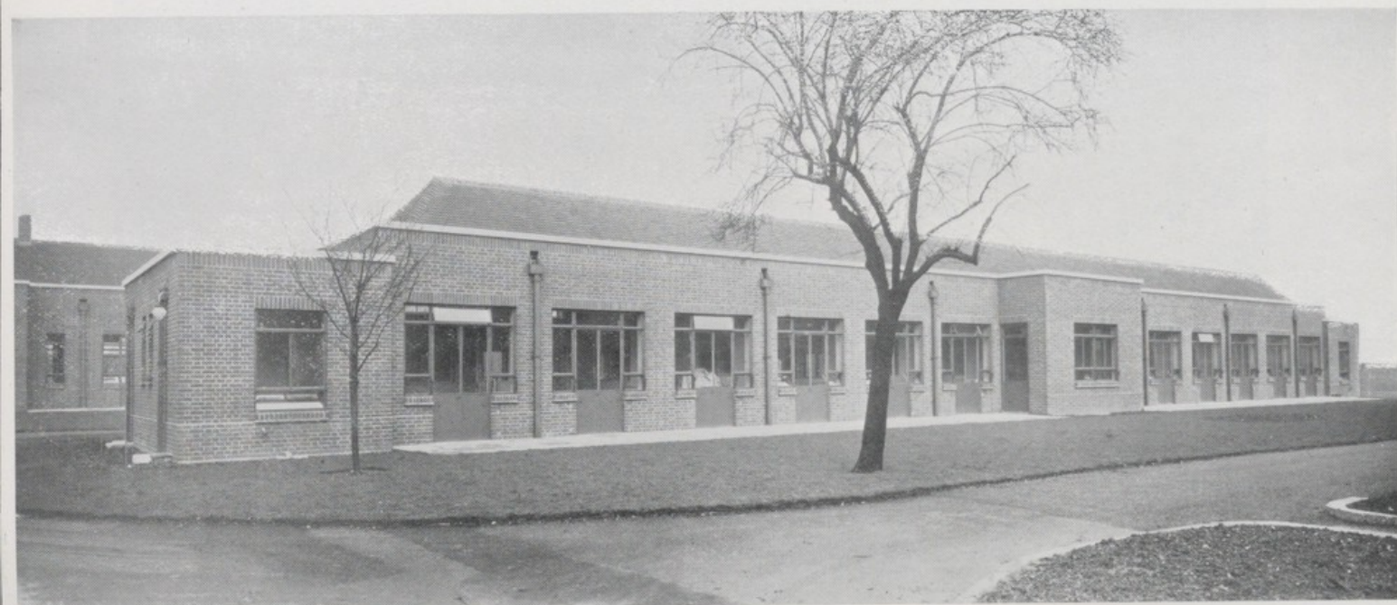
CLAYPONDS ISOLATION HOSPITAL CUBICLE BLOCK.
