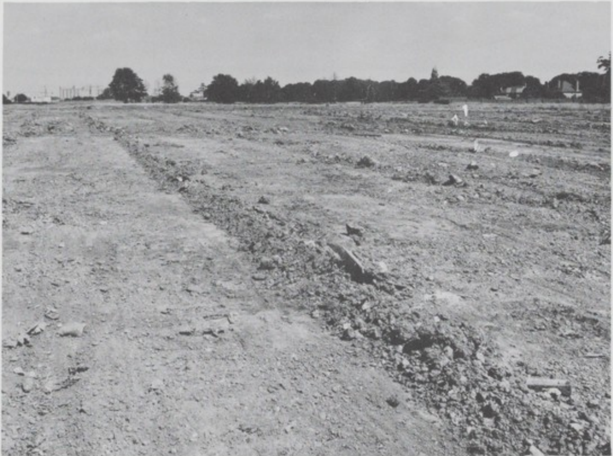
4. Covered, compacted and dressed ready for seeding
