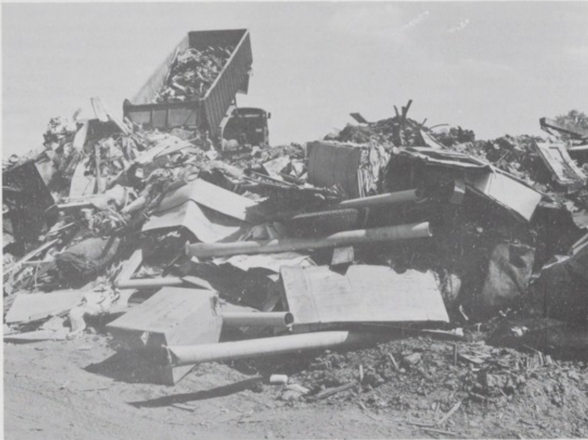
3. Rubbish tipped prior to covering
