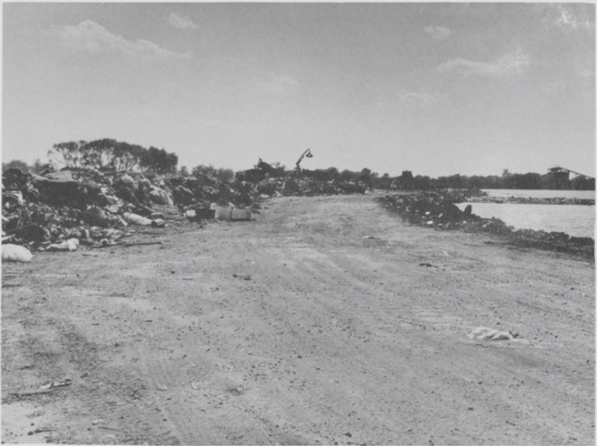
2. Road and base formed to receive rubbish
