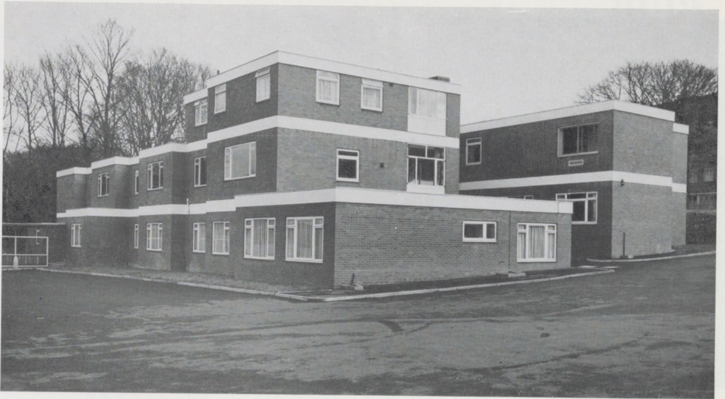
HURST ROAD HEALTH CENTRE (Opened June 1966)
