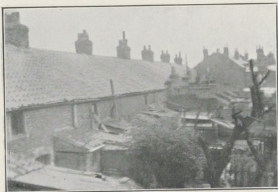
BILLET ROAD rear of Showing outbuildings and strutting to No. 4
