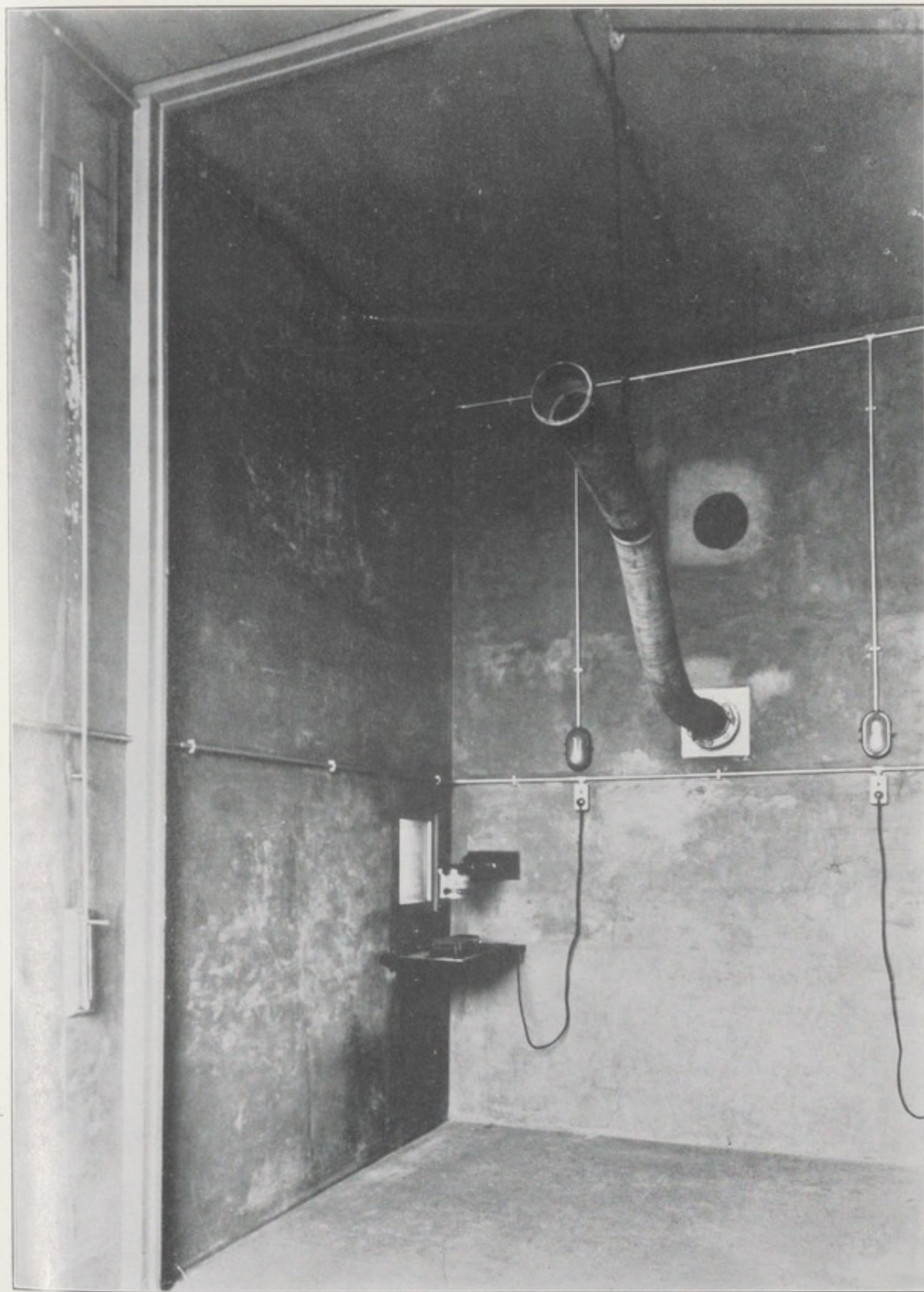
INTERIOR OF BUG DISINFESTATION CHAMBER SHOWING INSPECTION WINDOW AND TIN OPENER FACING SAME. THE TIN OPENING APPARATUS IS WORKED FROM THE EXTERIOR OF THE CHAMBER, THE TIN CONTAINING ZYKLON FUMIGATING MATERIAL. THE LARGE PIPE IS INSERTED IN THE FURNITURE VAN FOR EXTRACTING GAS AFTER FUMIGATION.
