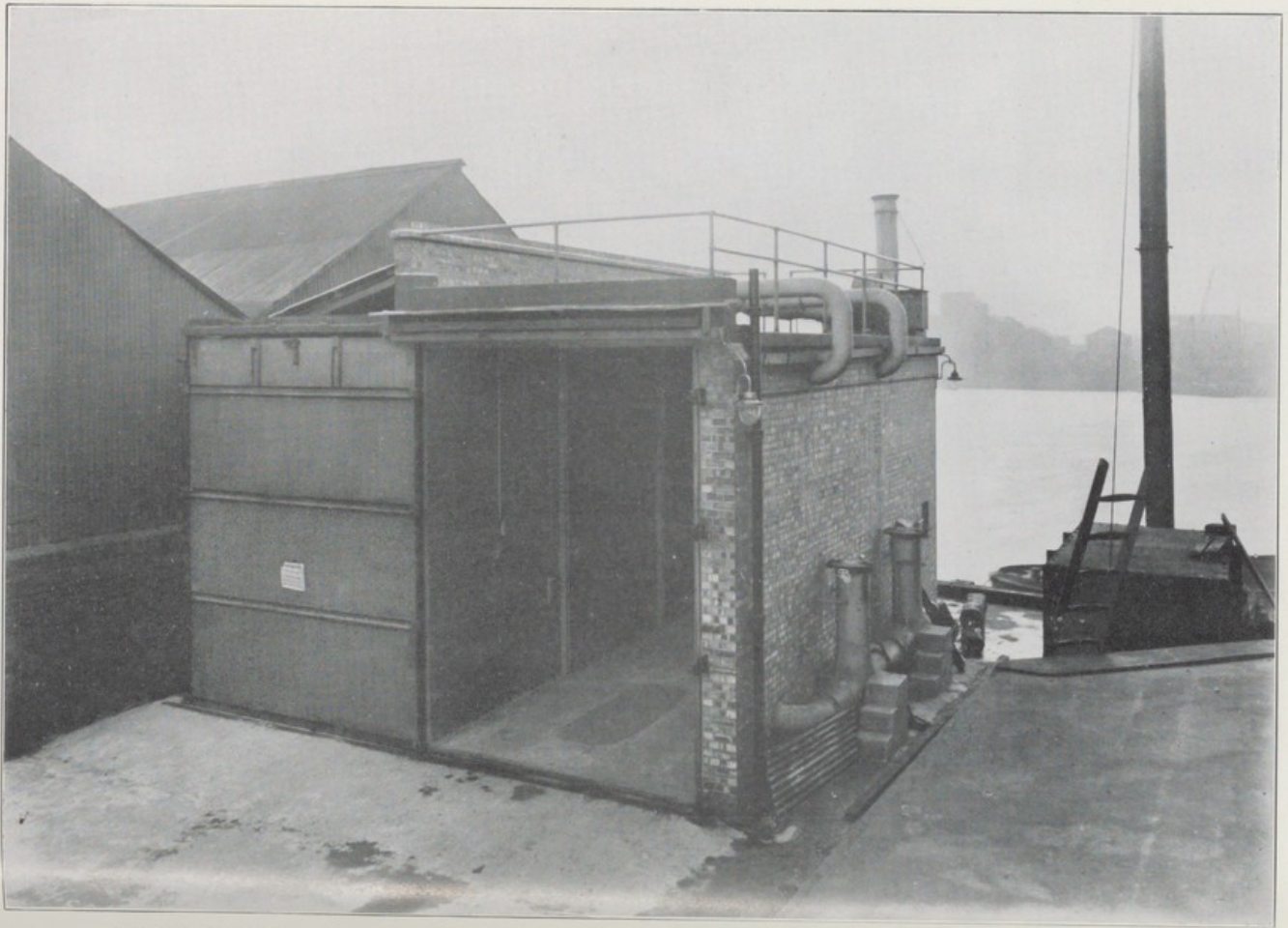
BUG DISINFESTATION CHAMBER FOR HYDRO-CYANIC FUMIGATION SHOWING EXTRACTION FAN AND AIR DUCTS. THE CHAMBER ACCOMMODATES FURNITURE VAN COMPLETE WITH FURNITURE AND IS FITTED WITH A GAS-TIGHT DOOR AND INSPECTION WINDOWS.
