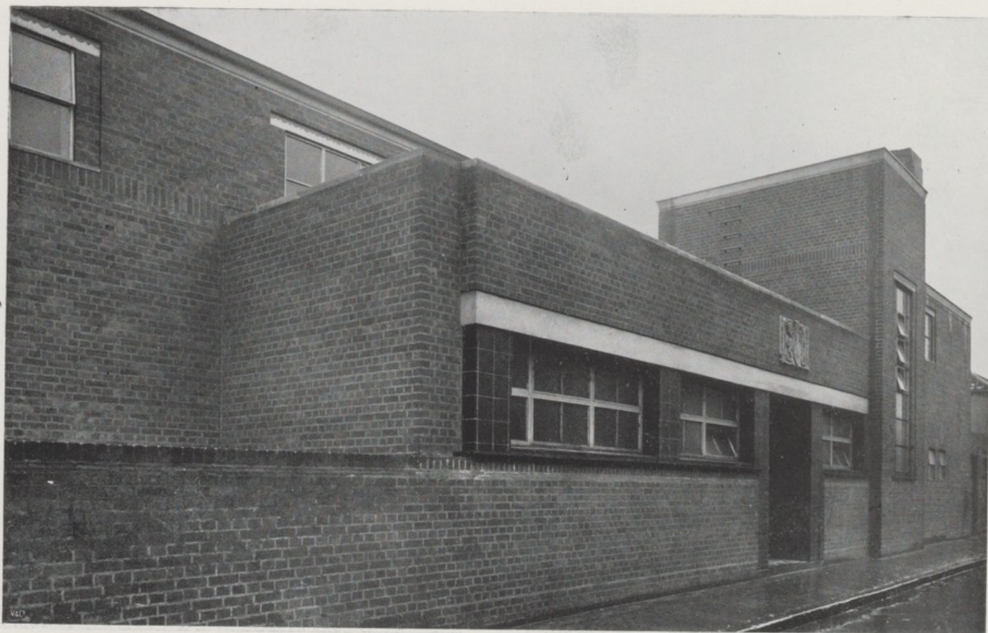
NEW TUBERCULOSIS CLINIC—ENTRANCE IN STEEL'S LANE
