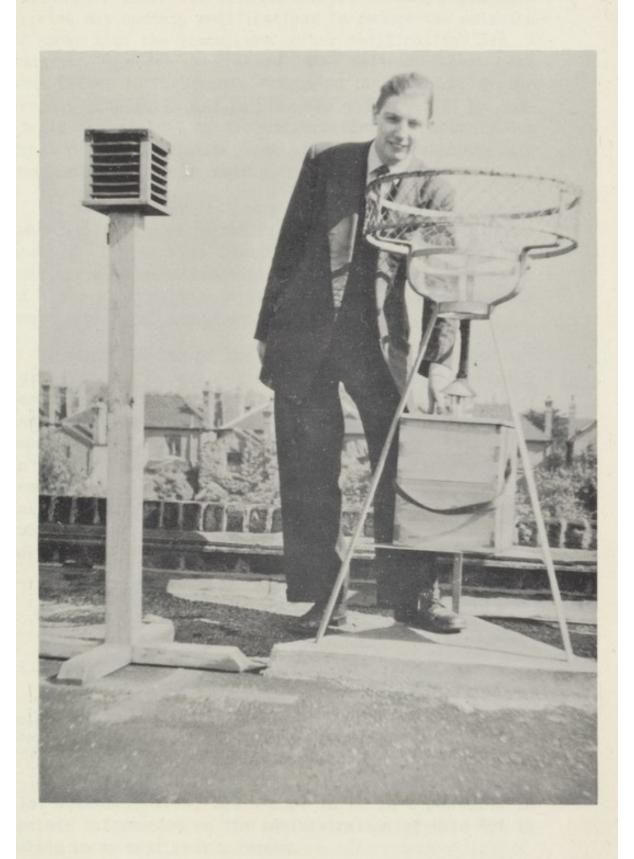
Deposit Gauge and Lead Peroxide Instrument at Longfield Avenue Depot
