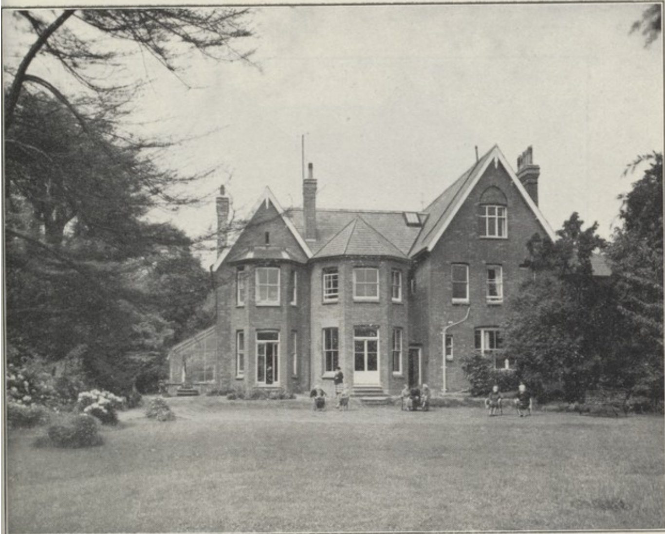
OLD PEOPLES HOME, "DOWNHURST," CASTLEBAR ROAD, EALING. (EALING EVENTIDE HOMES LTD).
