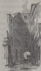
Entrance to Burgess' alley. (Looking out)
