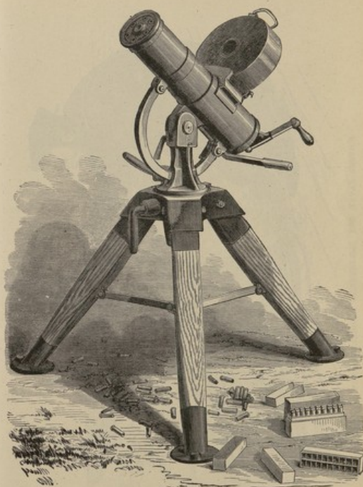
THE "PISTOL" GATLING, SIX BARRELS, WEIGHT 78LB.; CAPABLE OF FIRING 900 SHOTS A MINUTE.
