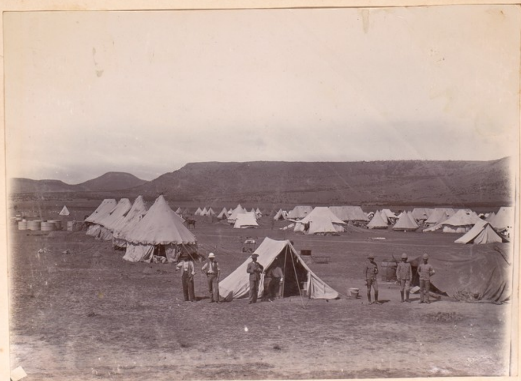
A part of Intombe Camp Hospital
