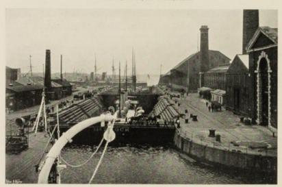
DOCKS No. 7 AND No. 10. Convertible into a single dock by removing the caisson
