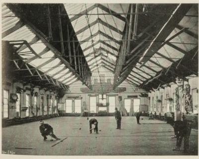
THE SHIP-BUILDING MOULD LOFT.
