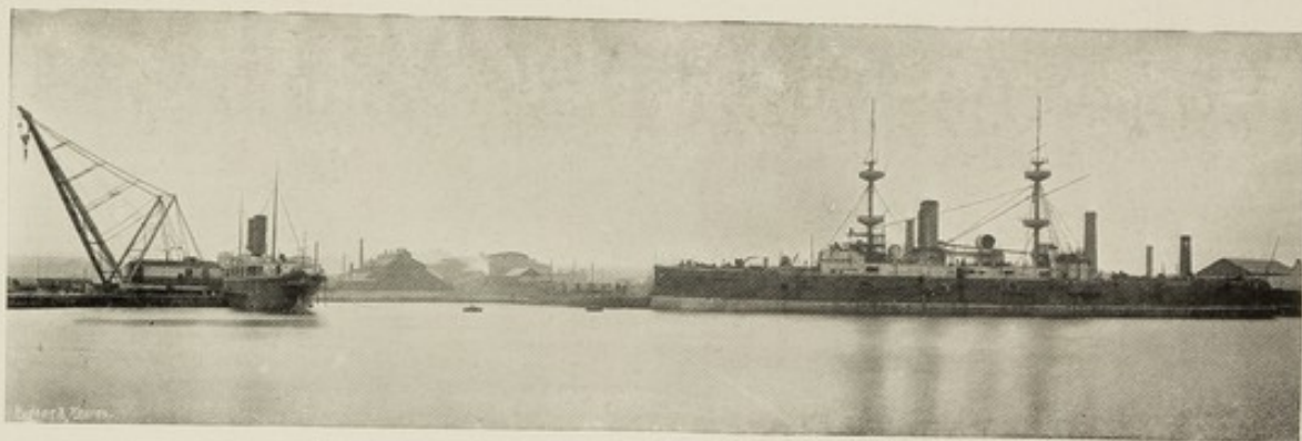
The Fitting-out Wharf at Messrs. Laird's, Birkenhead, showing the Boiler Shops and H.M.S. "Mars."
