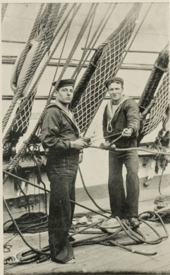
THE MODERN STYLE:—Serving a Wire Rope.
