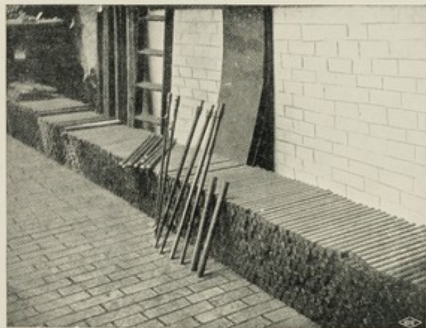
Rifle Barrels—Finished and Unfinished.
