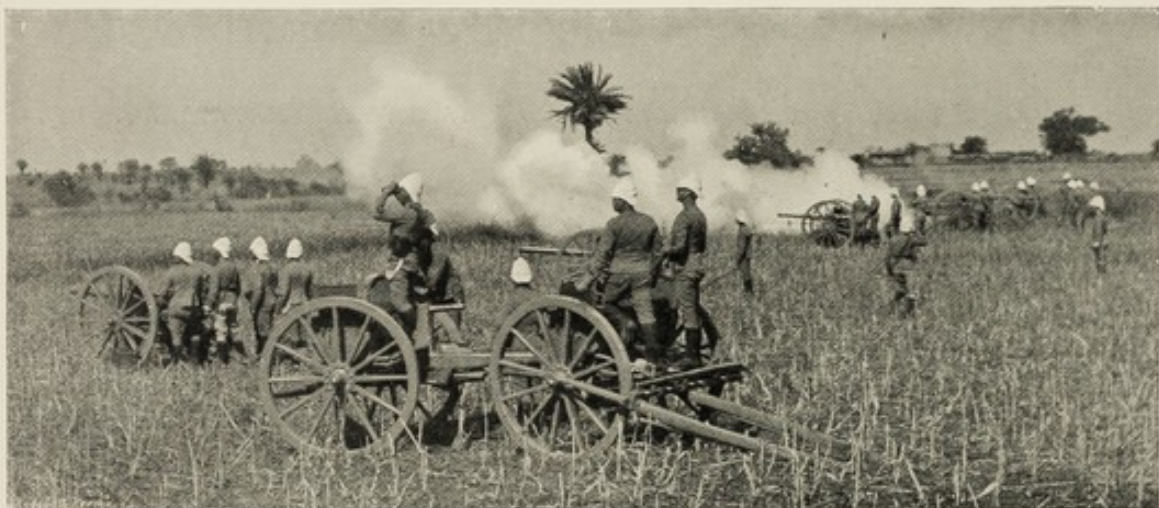
BATTERY IN ACTION.
