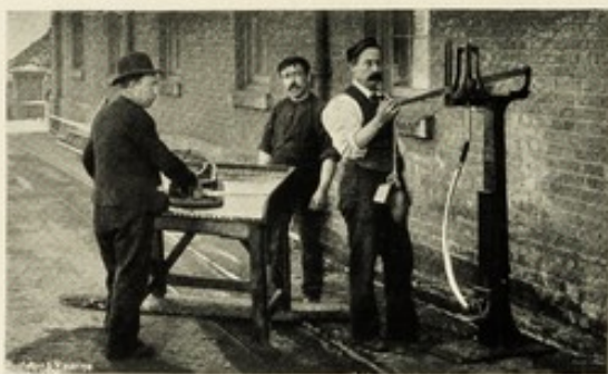
GUILTY OR NOT GUILTY? Good Steel or Bad. The Bending Test being Applied to Sword and Bayonet.
