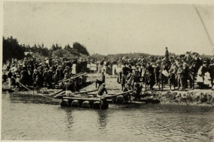
THE CANTERBURY ENGINEERS. Launching a Barrel Pier.
