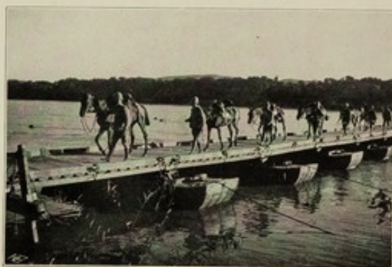
THANKS TO THE ROYAL ENGINEERS. An Excellent Pontoon Bridge.
