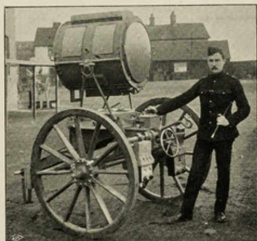
A SEARCH-LIGHT APPARATUS FOR FIELD USE. Equally Useful to Discover or to Signal.
