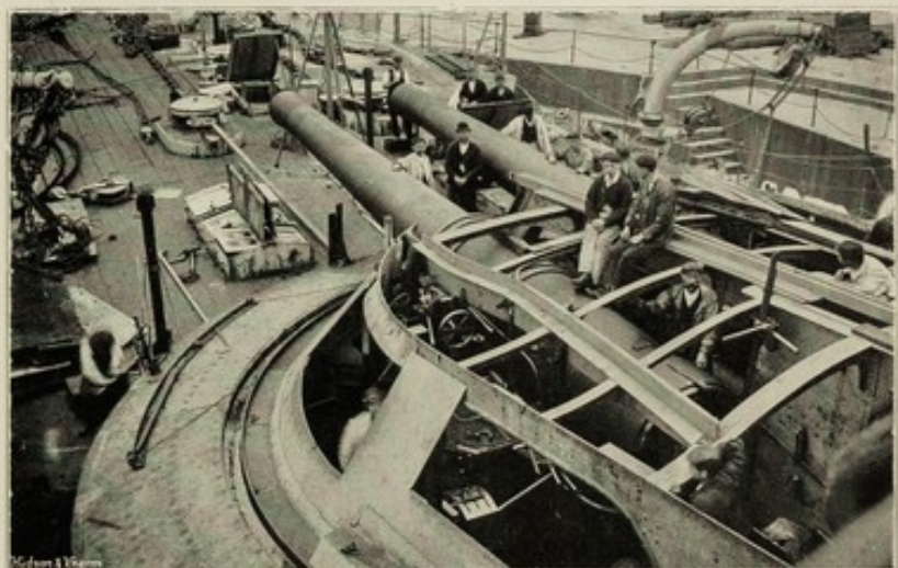
A BATTLE-SHIP'S BARBETTE NEARING COMPLETION.
