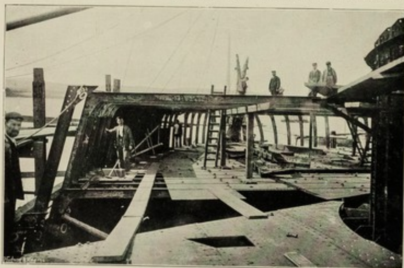
THE STOUT STERN OF AN ARMoured CRUISER. And the Bulkheads that Sub-divide the Hull.
