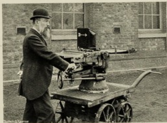
THE OLD ORDER GIVING PLACE TO THE NEW. Mr. J. Marks, Principal Manufacturing Foreman, Manipulating a Nordenfellt Machine Gun. Bore 1-in., Ejecting Steel Bullets Weighing 7½ oz.
