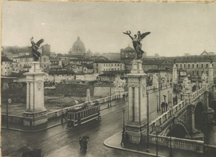
ROMA - Ponte Vittorio Emanuele. — The Victor Emanuel Bridge. — Pont V. Emanuel. — Viktor Emanuel-Brücke.
