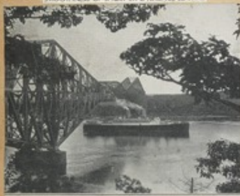
THE QUEBEC BRIDGE
