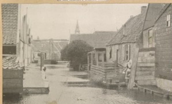
Land is so scarce in Holland that the pig-sty back of the second house on the right had to be built out over the canal on piles
