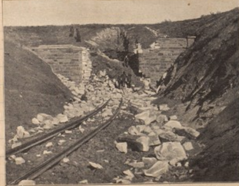
After the blowing of Almond's Nek the Boers evacuated Laing's Nek and Majuba. When our men reached Laing's Nek, about 100 yards each end of the tunnel were found to have been blown in by the enemy. The debris was lying about in heaps, but the line was otherwise unaltered. Our photograph is by J. Ferguson.
