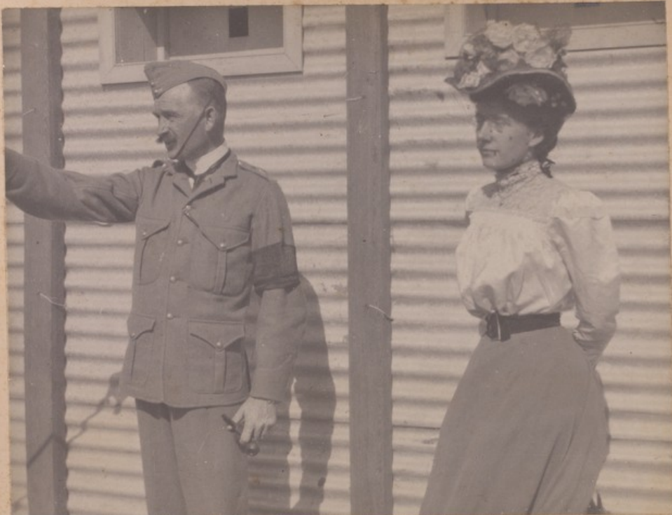
Col. Woodhouse and Ethel. Outside a blockhouse. East London. 1901
