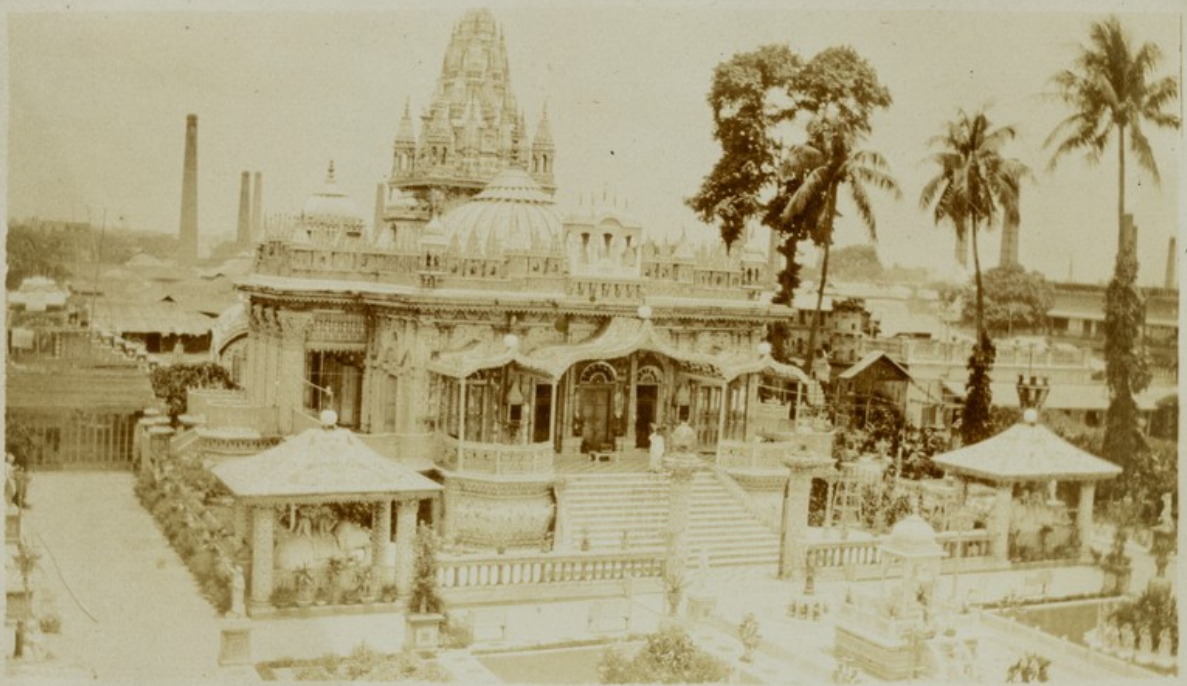
No. 22. ANOTHER VIEW TAKEN FROM LEFT SIDE.
