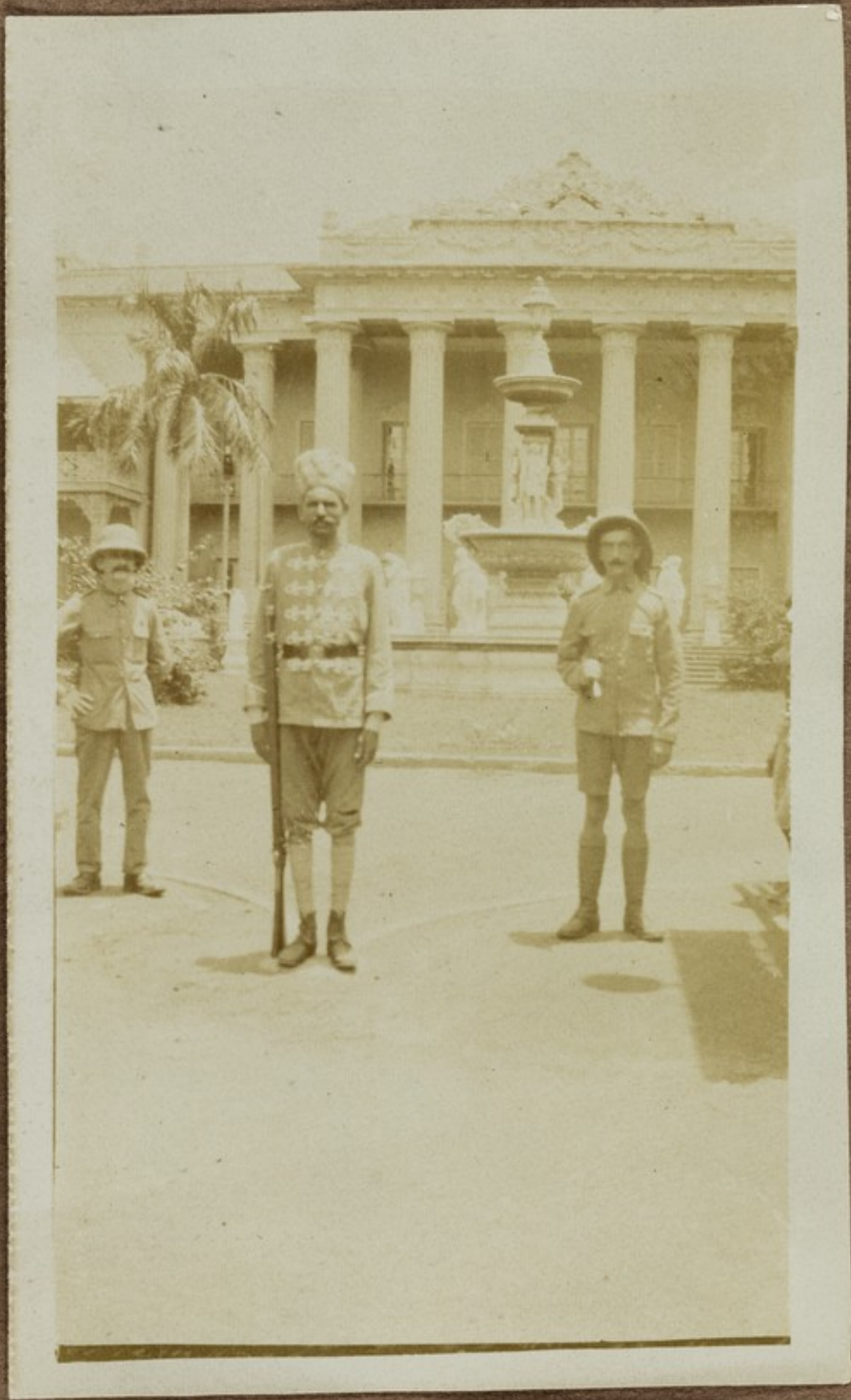
NO 26 ENTRANCE TO THE MARBLE PALACE, CALCUTTA OWNED BY SOME WEALTHY JAIN.
