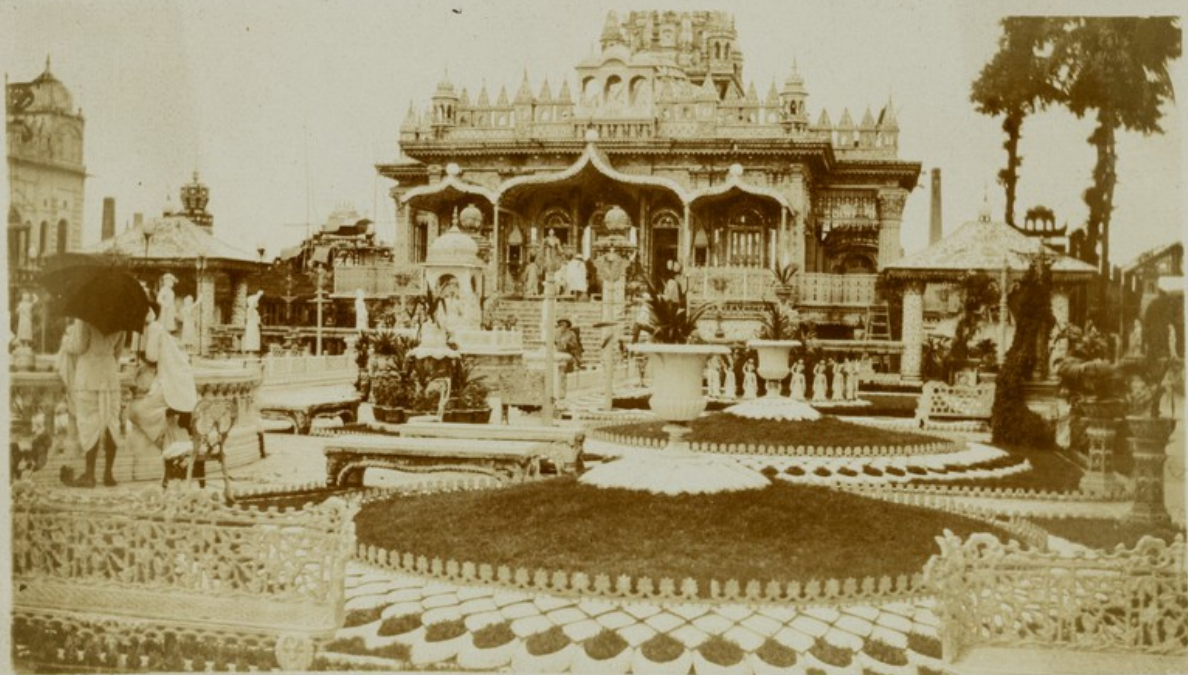
NO. 21. FRONT VIEW OF TEMPLE TAKEN INSIDE THE GROUNDS.
