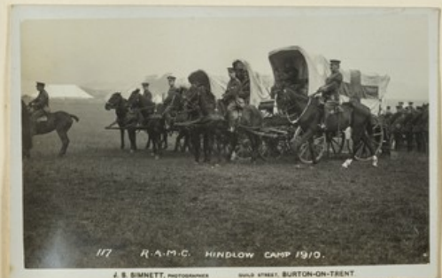
2 ND N. MID. F. AMB. R.A.M.G. Inspection
