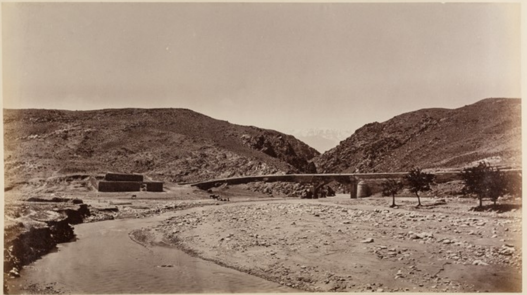
Surath- and bridge showing barge
