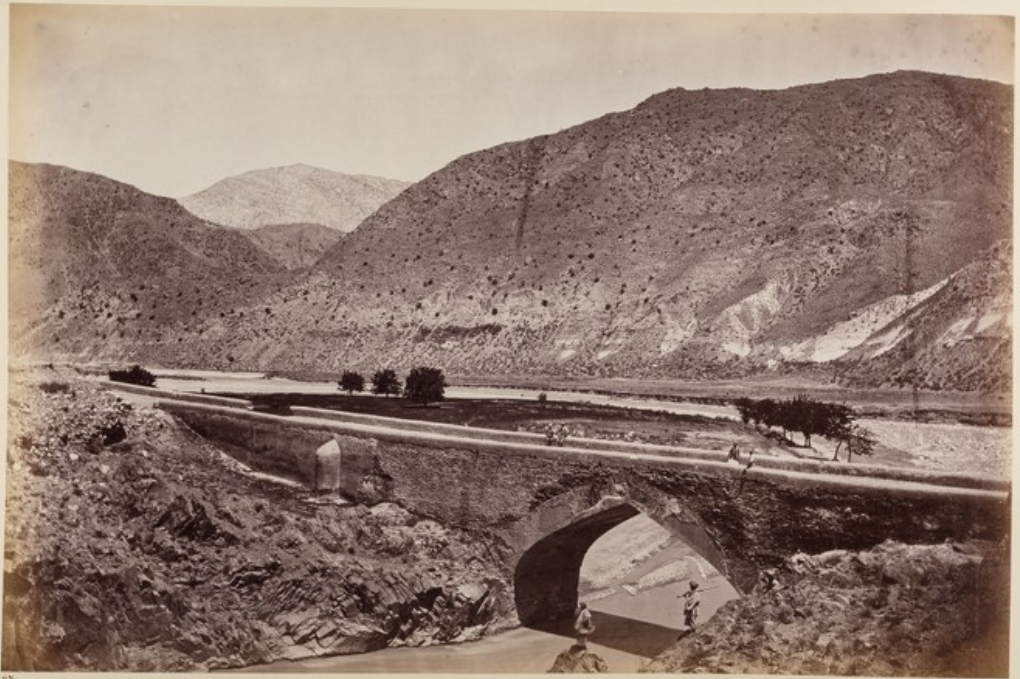
Sivakoti, Nepal, The bridge from the gorge looking down stream
