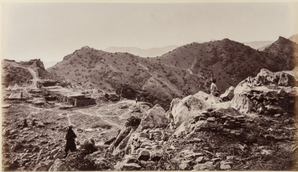
View looking up western wall of Fort, showing right corner bastion and position of the three conical peaks forming enemy's right defence with entire line of Sunya.
