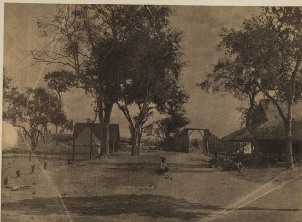
The East Gate of Bhamo. 1886. Inside the Stockade.
