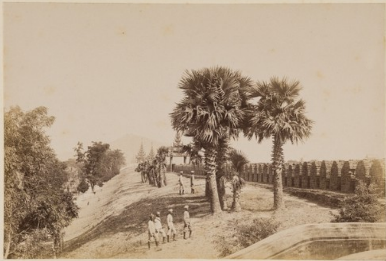
Earthwork inside the City Walls.
