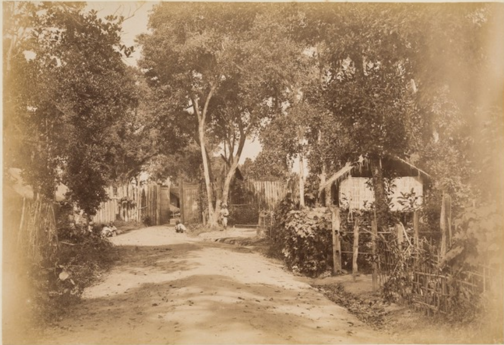
South Gate of Bhamo.
