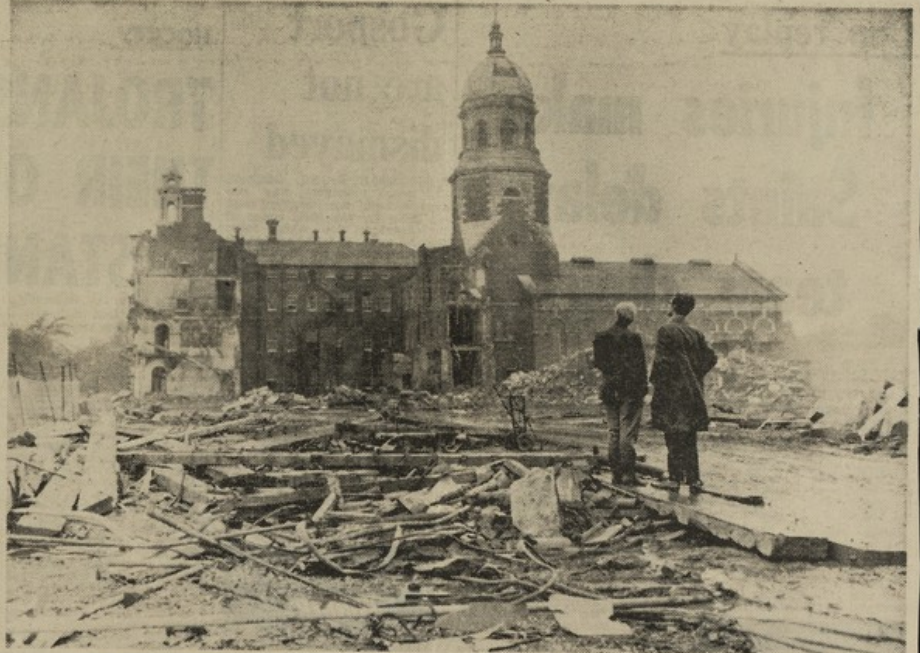
Part of Netley hospital still stands. In the foreground, a tangle of old pipes and debris.—"Echo" photo.
