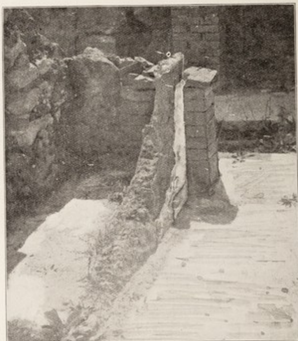
FIG. 8.—REMAINS OF THIN PARTITION WALL OF CLAY CASSED WITH PLASTER— S.E. QUARTER. (The wall has been supported by modern brick piers to preserve it.)
