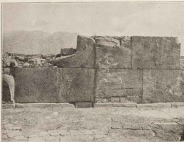
FIG. 6.—LIMESTONE MASONRY: CENTRAL COURT, PILESTOS.
