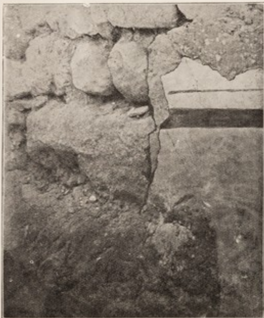
FIG. 7.—WALL OF THE THIRTEENTH MAGAZINE, KNOSSOS, SHOWING THE METHOD OF FINISHING RUBBLE WALLS WITH PLASTER.
