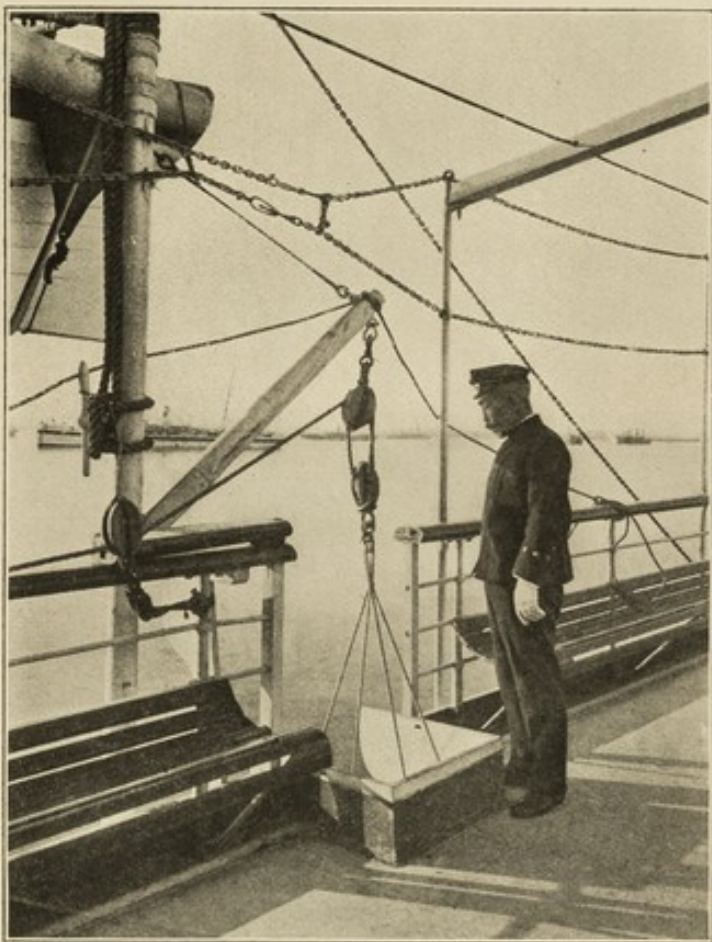
SAIKYO-MARU, SERIES NO 3. HATCH DEVICE ON HURRICANE DECK FOR HOISTING PATIENT ABOARD SHIP.
