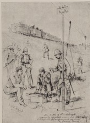
TAPPING THE TELEGRAPH-WIRE, ELANDSLAAGTE. Sketch (Facsimile) by our Special Artist, Mr. Milton Prior.
