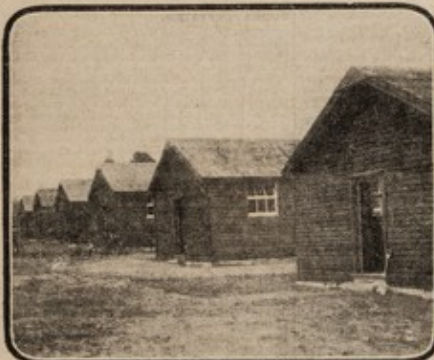
The new wooden huts. They are lined with asbestos and lighted by electricity. —(Daily Mirror photograph.)
