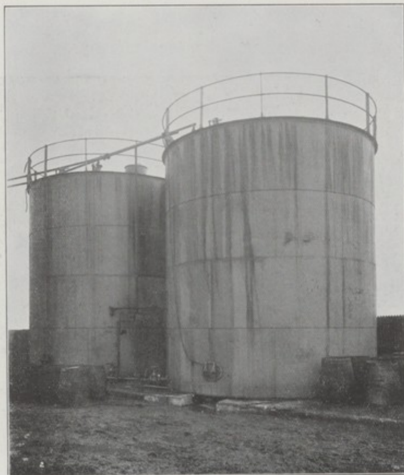
TALLOW STORAGE TANKS.
