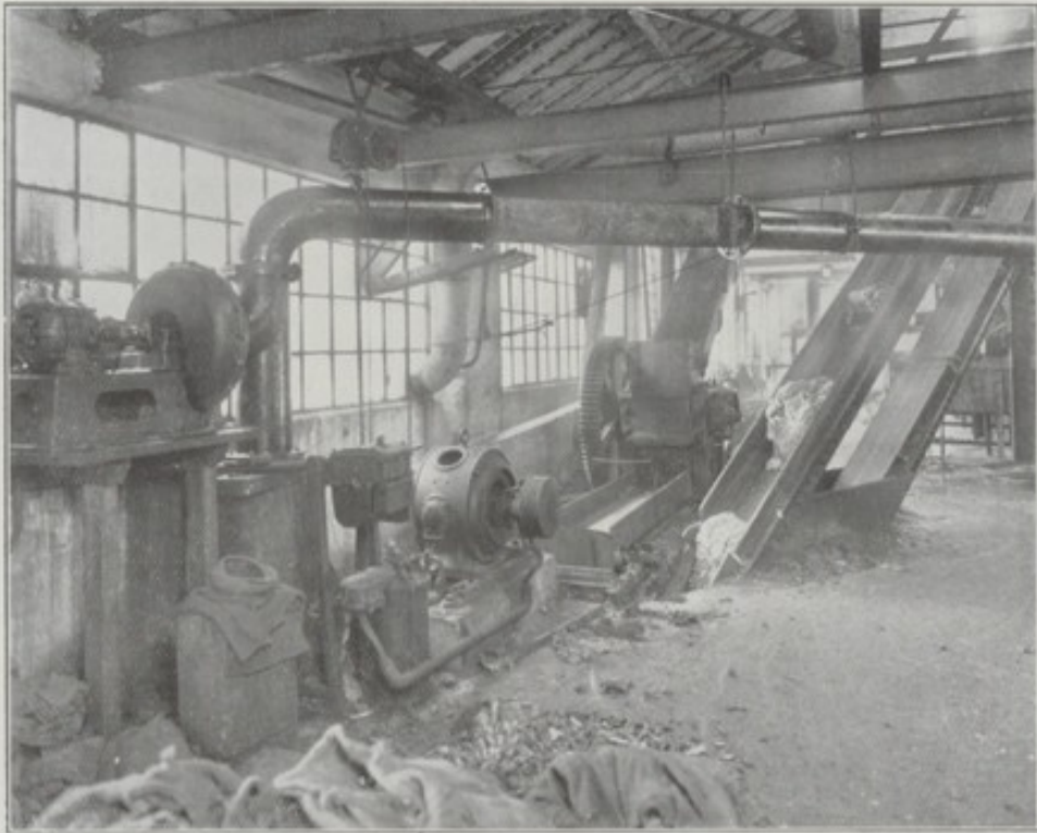
CRUSHER AND ELEVATOR.
