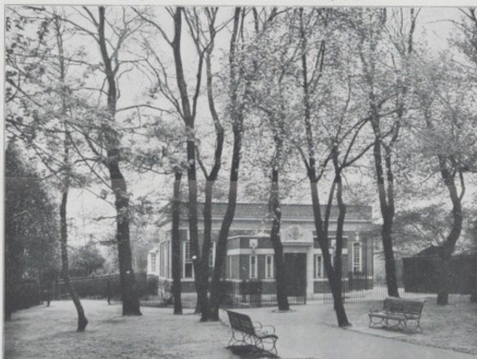
Hornsey School Clinic Exterior, taken from Broadway Gardens.
