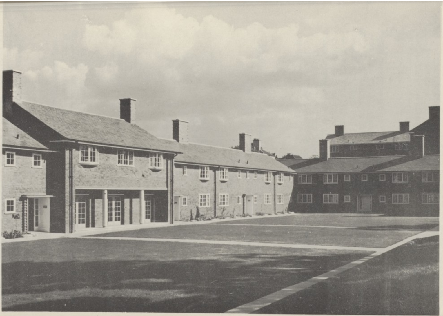
ALMSHOUSES - Sycamore House, Sycamore Gardens.
