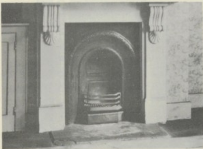
Open fire with gas ignition and new 6-piece brick set fitted in cast iron register grate.
