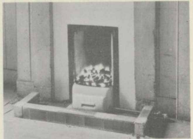
Open fire with gas ignition fitted in place of stool bottom grate.
