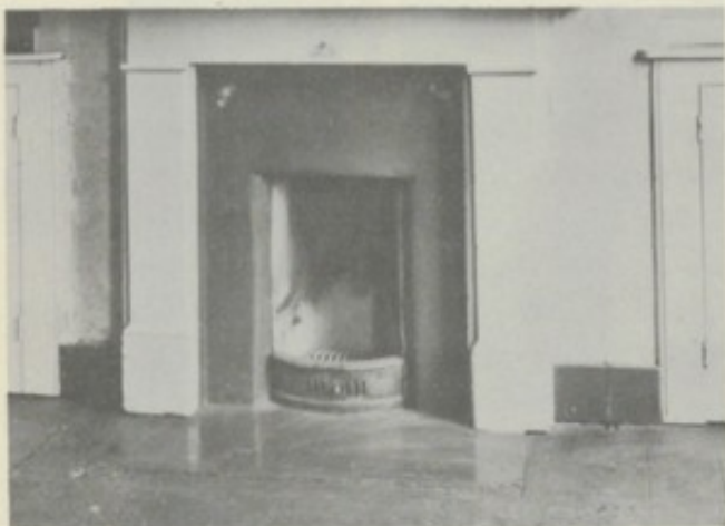
Fire opening filled in and convector type gas fire fitted.
