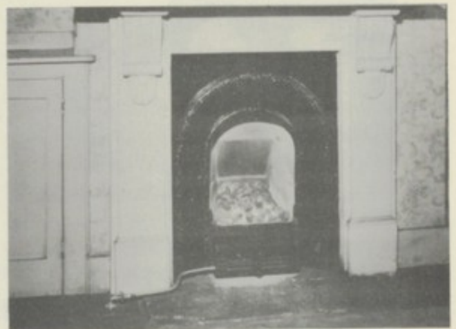
Open fire with gas ignition and new 6-piece brick set fitted in cast iron register grate.
