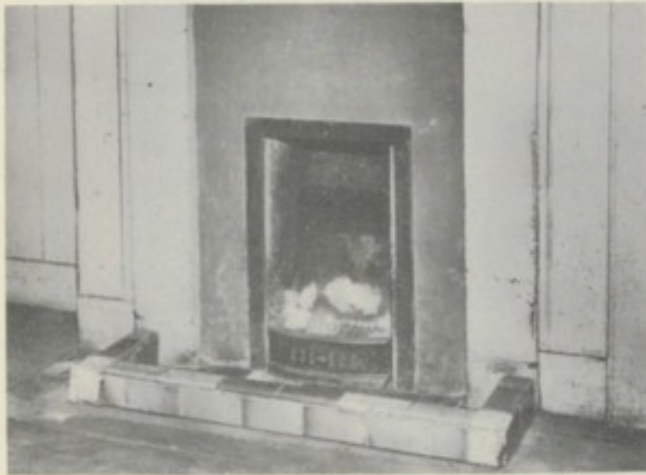
Open fire with gas ignition fitted in place of stool bottom grate.
