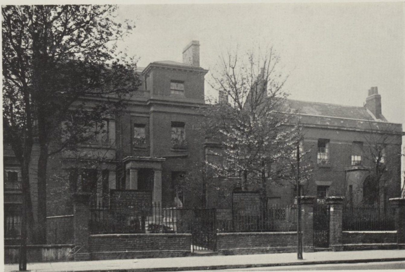
THE ORIGINAL GRANGE ROAD WELFARE CENTRE AND T.B. CLINIC, 1934. NOS. 108-110 GRANGE ROAD
