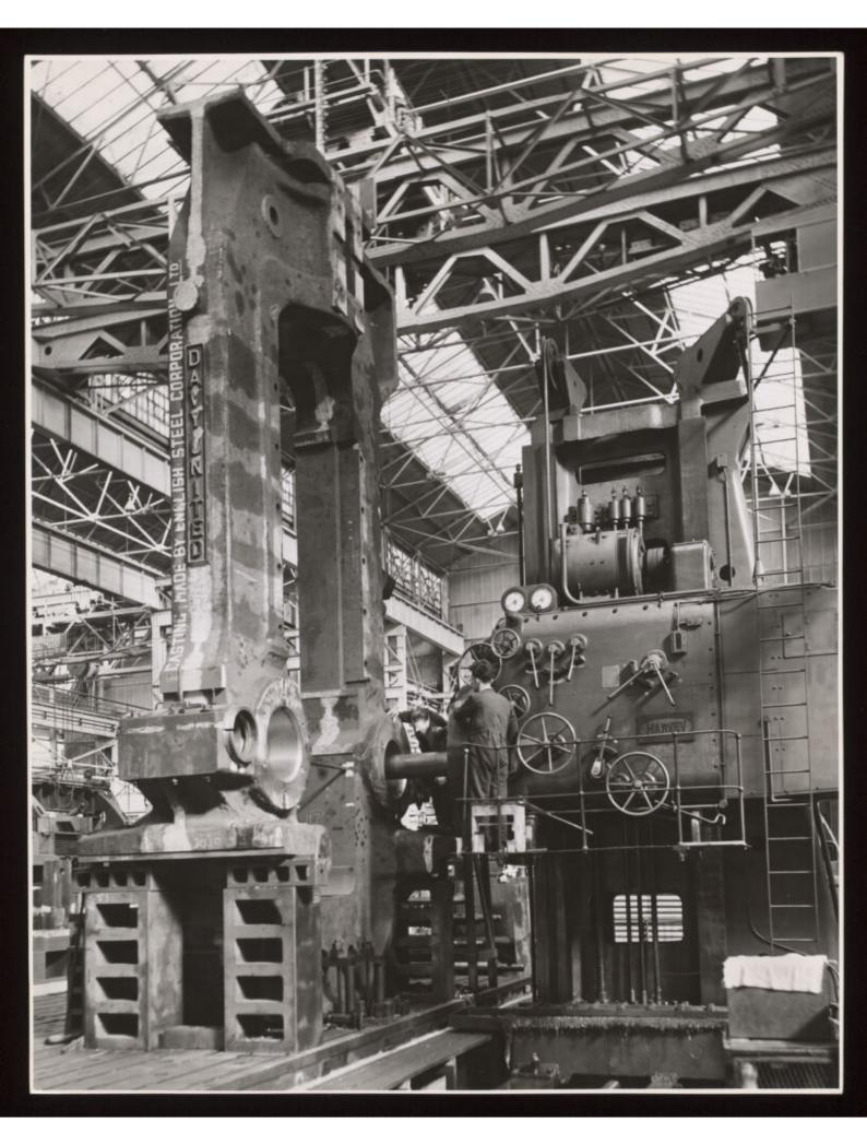
Engineering shop conditions in the firm of Davy and United Engineering Company, Ltd., Park Iron Works, Sheffield 4. One of a series of fourteen photographs supplied by Mr. F.R. Smith, Publicity Officer, 17th January, 1957. No. 3366. Modern heavy machining conditions. The machining of a 100 ton roll housing for a heavy slabbing mill on the large type horizontal boring, milling and drilling machine which is now used a great deal in shops of this capacity.
