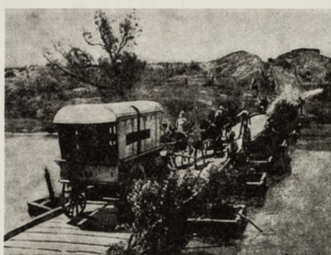
Surgeon-Major Beevor took this photograph of an ambulance crossing the Modder River on a pontoon built by the engineers as the British advance against the Boers.
