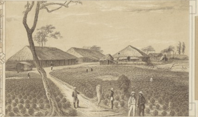
NEW STATION, ROSEKANDY, COOLIE LINES ASSAM.
