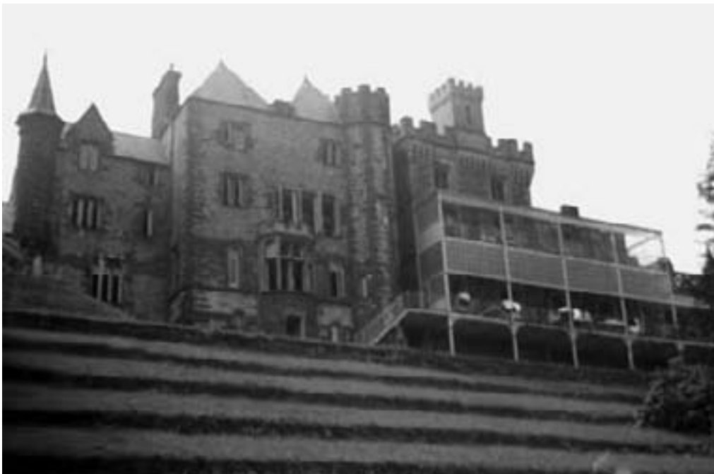
Balconies at Craig-y-nos. These were built when the castle was converted to a sanatorium. They were roofed and the sides were glazed but until the 1950s the fronts were open to the elements. Courtesy Mari Friend.
