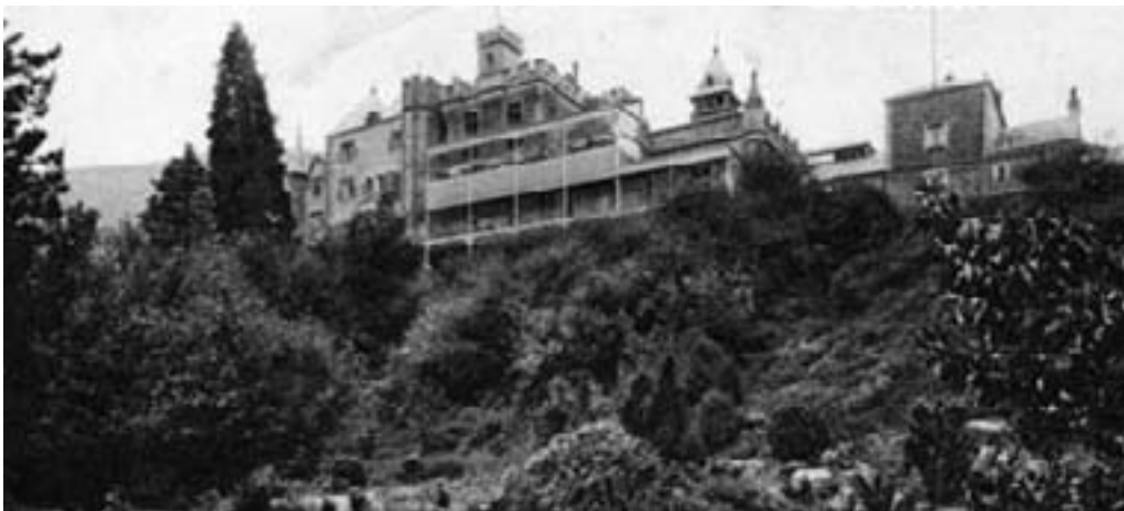
The balconies from the rockery. Some patients and staff experienced inexplicable events or impressions, both within the buildings and grounds. From a postcard, 1950s.
