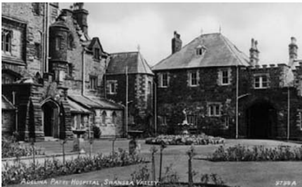
In this view of Craig-y-nos, the main entrance door is left, whilst the buildings behind the fountain (centre) housed the X-ray and light therapy rooms, operating theatre and dental department. From an old postcard.
